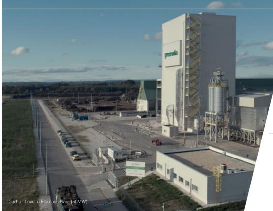
The plant is constructed on a plot of 103,000 square metres and has an installed power of 50MW, that can generate up to 375 GWh per year from forest biomass collected in the mountains in the region. The plant can treat over 500,000 tonnes of remains from forest thinning, from sustainably-managed plantations.
